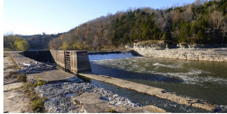
Kentucky Lock and Dam No. 11 | Rye Development
